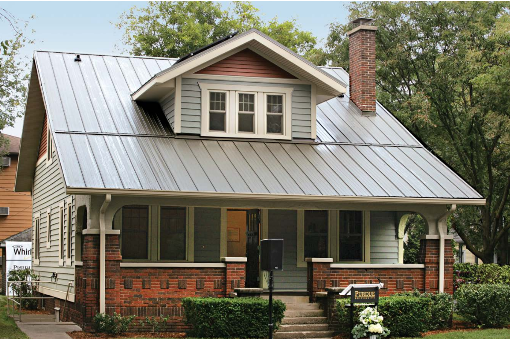
The ReNEWW House project began in April 2014 and will provide the foundation for developing super-efficient, connected appliances of the future.
