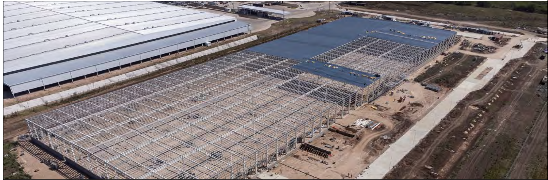
New manufacturing plant under construction in Argentina.
