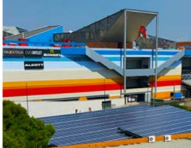
The Naples plant in Italy has a photovoltaic plant producing more than 630,000 kWh per year (approximately 10% of its electric needs), which brings a yearly saving of approximately 500 tons of CO 2 .
