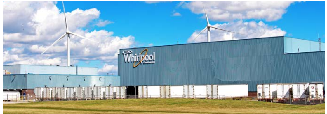
For more information: http://www.whirlpoolcorp.com/whirlpool-corporation-announces-plans-to-use-wind-turbines-to-power-findlay-ohio-facility/
